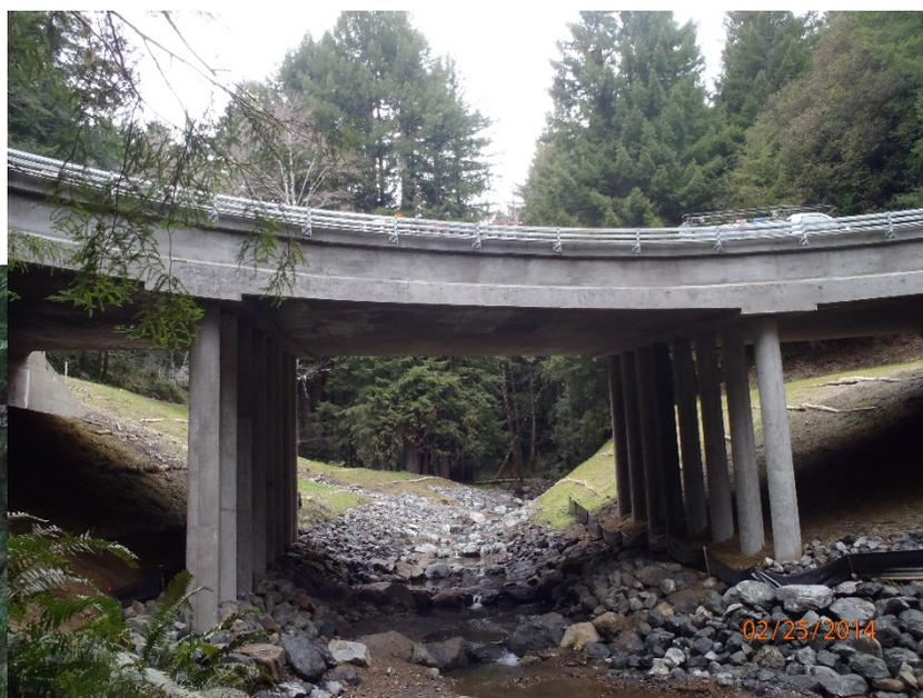
The 134-foot slab bridge (top photo) replaced a nine-foot steel plate pipe culvert that created a six-foot vertical drop and barrier to fish passage downstream. Photo credits: Caltrans (top).
