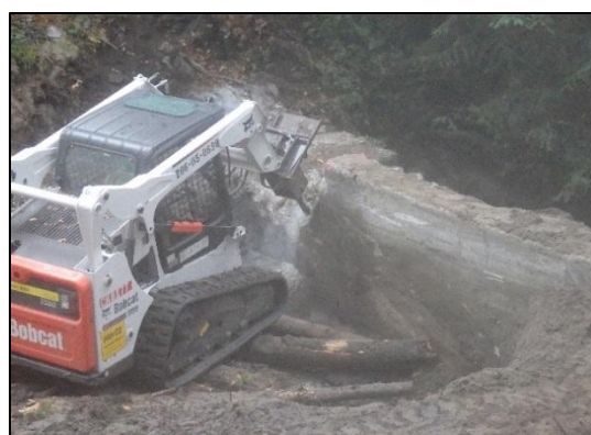
Figure 3. Bobcat chipping away at dam structure
