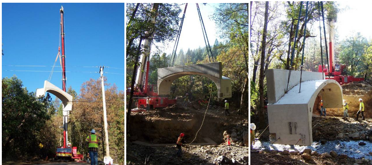
Above Placing the ConSpan arches on the footings
