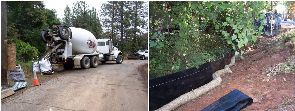
Above left concrete washout stations were required and riparian sediment fencing and silt waddles in place (right)
