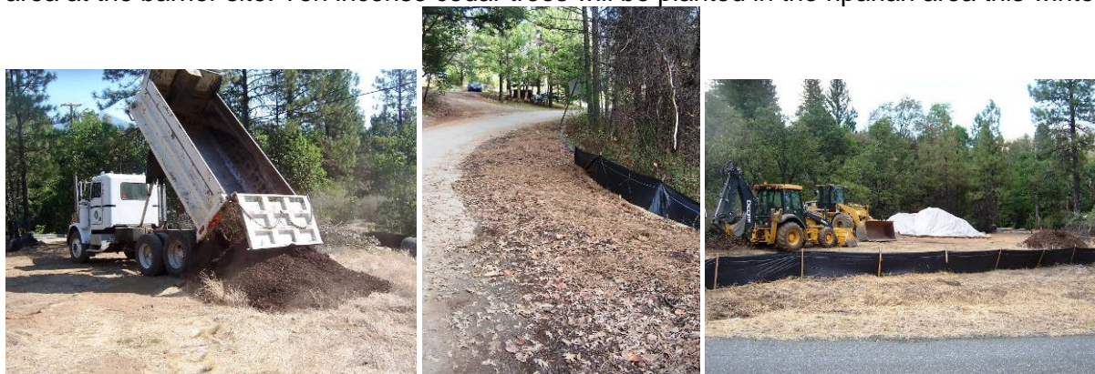
Organic compost (left) and native pine needle mulch (middle) were applied and water quality BMP's applied (right).
