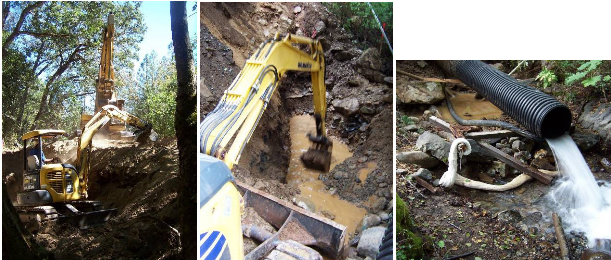
Excavating channel (left) and footings (middle) and water quality protections during jetting, which created the most turbid water conditions (right).
