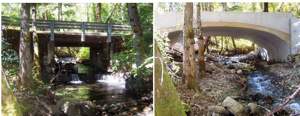
Conner Creek Road Project Before with 10' concrete box culvert looking upstream (left) and restored channel with 24' wide bridge (right).
